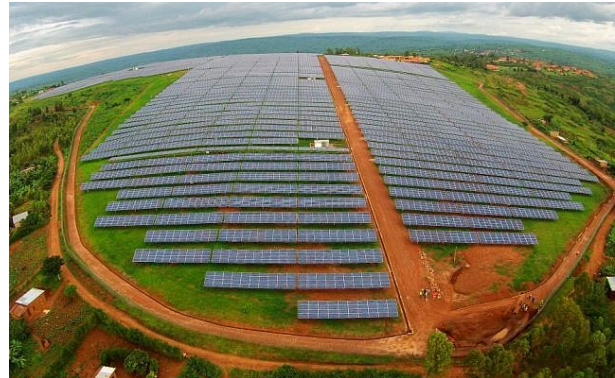
Figure 3. Utility-scale of 8.5MW PV power plant constructed in Agahozo-Shalom Youth Village in Rwanda
