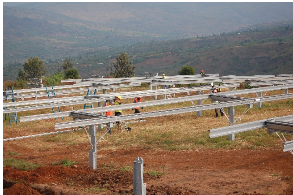
Figure 8. CPP under Construction in the cafeteria at the Agahozo-Shalom Youth Village
