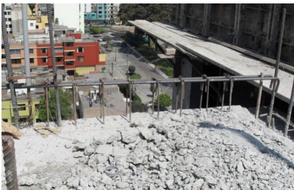
Figure 16. Reinforcement of an unfinished cambered beam
