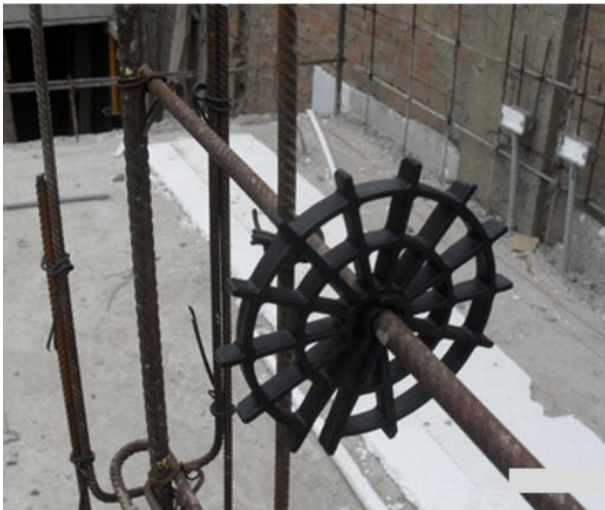
Figure 11. Polymer-based spacer for the steel reinforcement of vertical concrete elements
