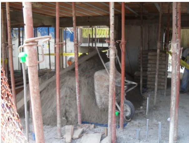
Figure 23. Construction materials accumulated on the construction site
