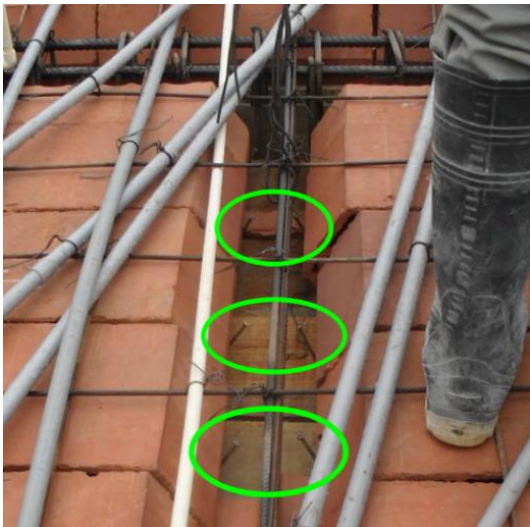
Figure 19. Method for fixing ceiling bricks
