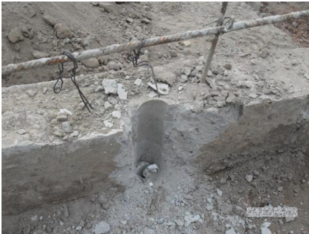
Figure 6. Partially poured concrete wall
