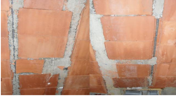
Figure 18. View from beneath a lightweight slab
