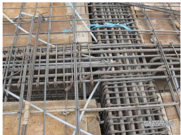
Figure 15. Reinforcement congestion in a beam frame
