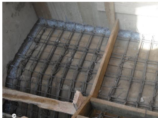
Figure 8. Concrete walls next to the stair landing, roughly hewn horizontally
