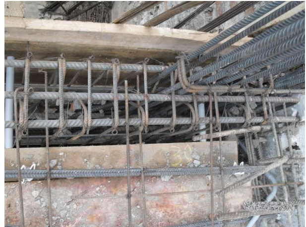
Figure 14. Intersection of beam and column reinforcement
