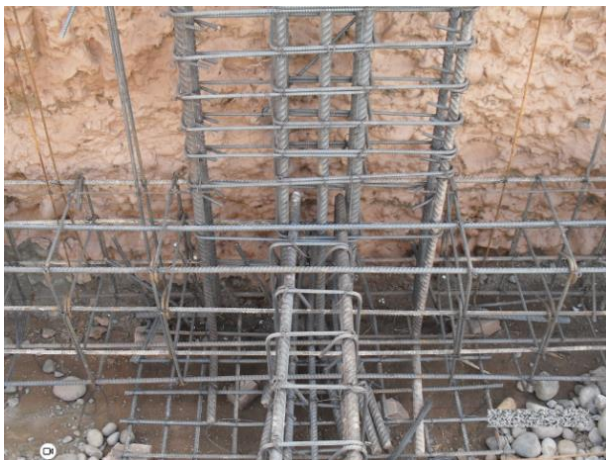
Figure 5. Footing prior to pouring without screed
