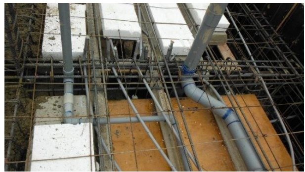
Figure 21. Wall-mounted drain battery
