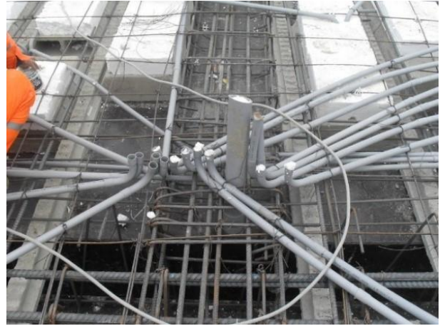
Figure 20. Clustering of pipes in a solid slab
