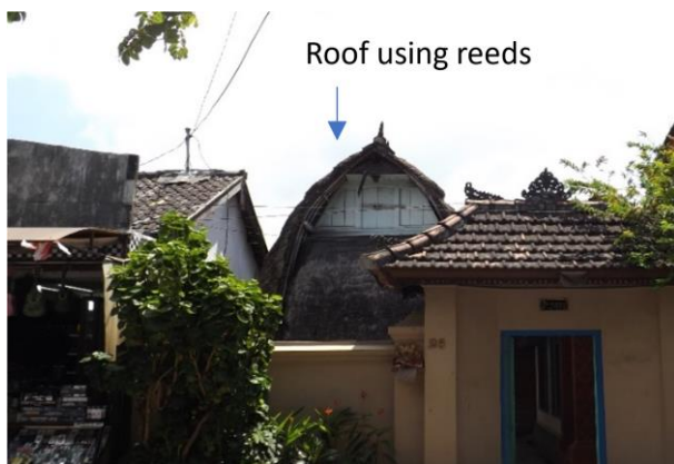
Figure 3. Reeds and palm fibre for the roof of Balinese buildings in Kuta
