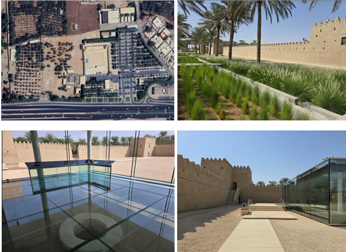
Figure 4. Qasr Al-Muwaiji, Al Ain: After restoration and sustainable/desert landscape referencing the falaj irrigation system (Images by authors and google maps)
