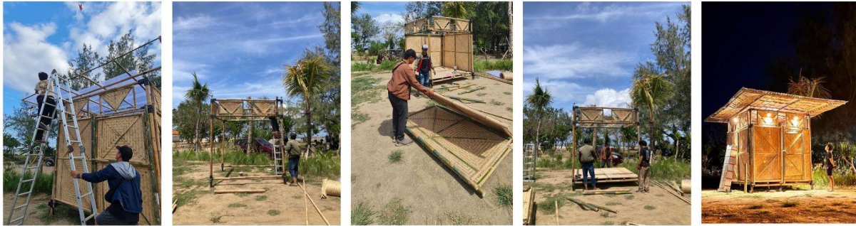
Figure 8. The field assembly of the prefabricated bamboo cabin prototype
