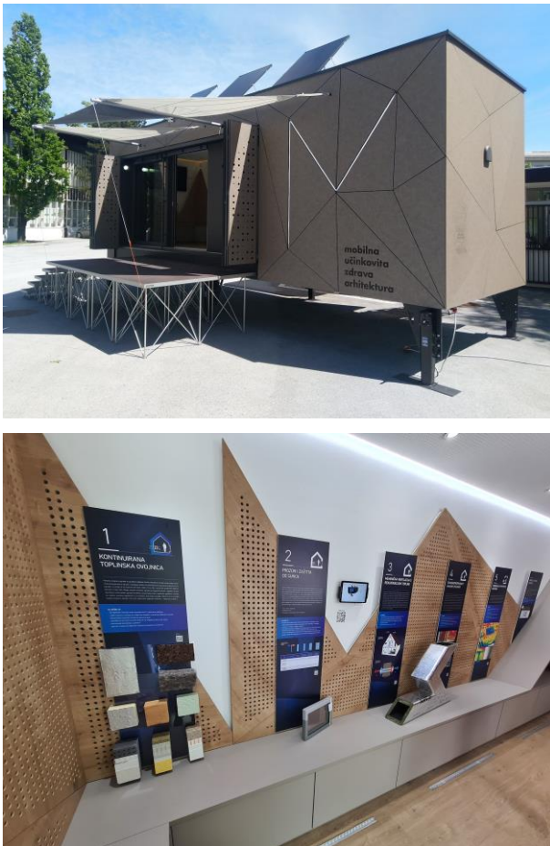
Figure 11. Living Laboratory (a exterior, b interior) – Mobile Nzeb house (Project Manager: B. Milovanović) called MUZA (Mobile Efficient, Healthy Architecture) – resting construction according to NZEB standards, where visitors will be able to learn about NZEB and experience NZEB first-hand. MUZA conducts measurements of indoor environmental quality parameters, such as temperature and relative humidity, CO 2 concentrations in the air, relative air quality, and measurements within the layers of the building's outer envelope, Zagreb, 2021, Authors: N. Vezilić Strmo and M. Sladoljev (source: author's archive)
