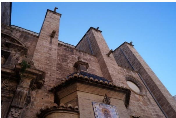
Figure 7. Buttresses of Los Santos Juanes
