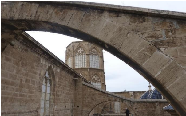
Figure 6. View of the flying buttresses of Valencia Cathedral [10]
