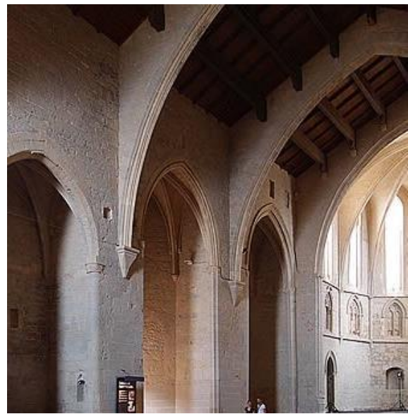
Figure 2. Convent of San Francisco de Morella. The accompanying figure shows the construction of the wooden roof [9]
