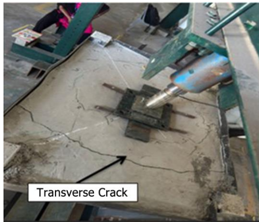
Figure 13. Crack Pattern of Infilled Composite Frame
