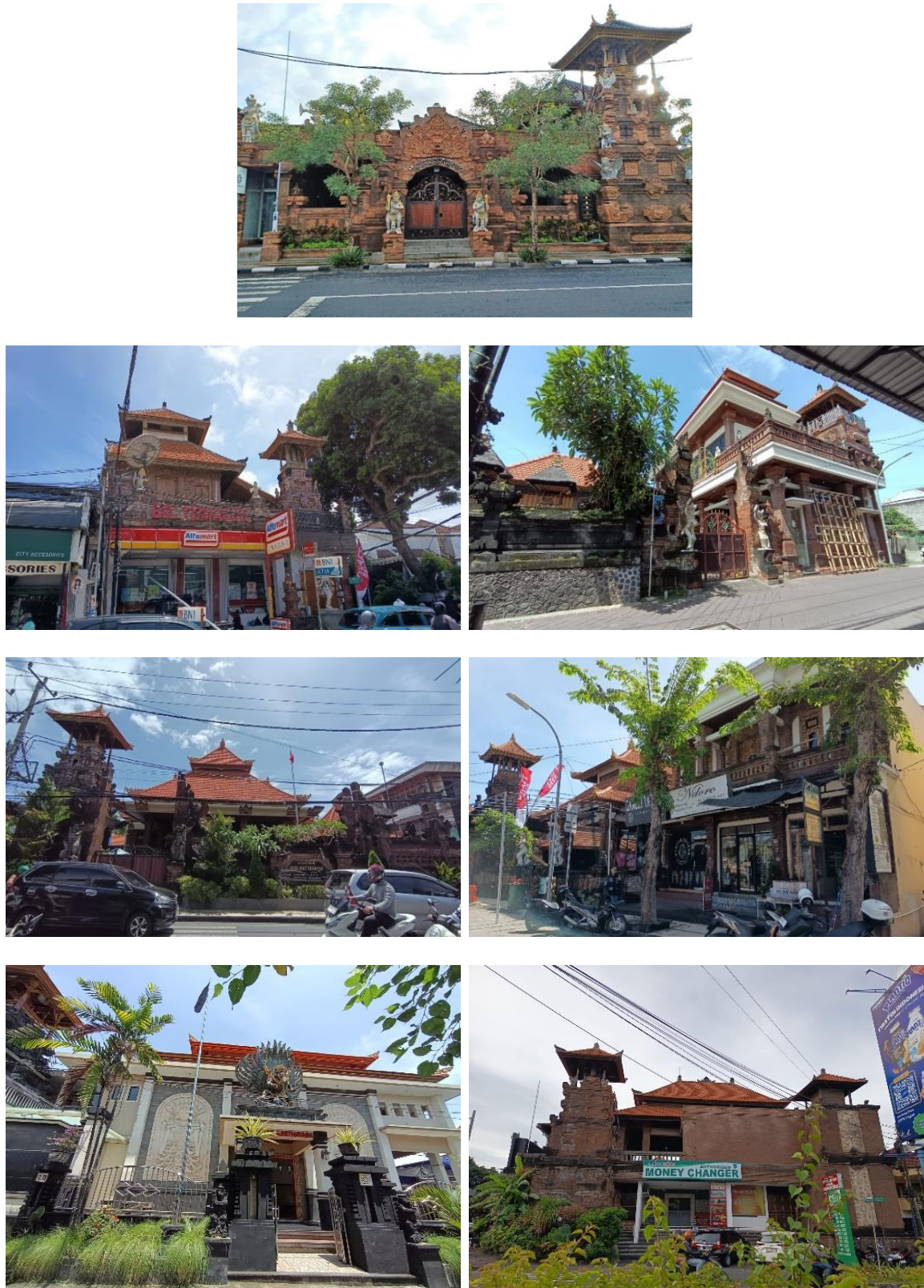
Figure 4. Visual Contrast of Traditional Bale Banjar Architecture and Modern Bale Banjar Renovation in Kuta. Source: Field Documentation, Researchers, 2025
