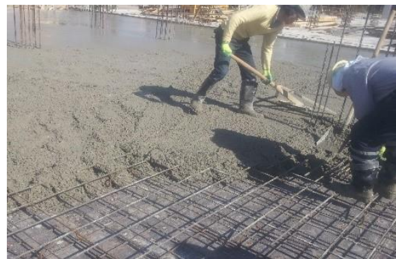
Figure 1. Pouring concrete for a monolithic inter-floor slab
