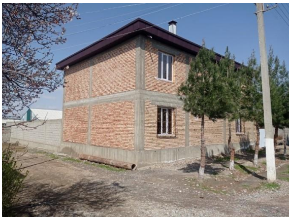
Figure 2. The exterior of an existing residential building
