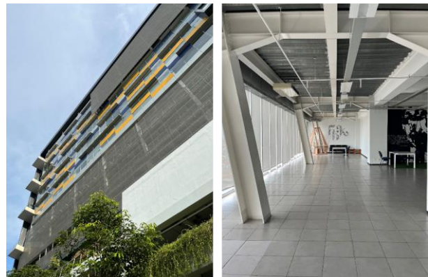
Figure 1. Facade and interior of the Q Building Gallery
