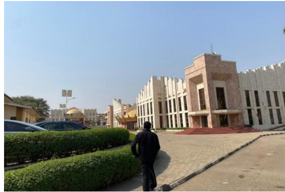
Plate 1. Front Facade of Family Worship Centre Building (Author's Fieldwork, 2025)
