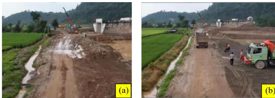
Figure 6. Visual results of field stabilization tests: (a) existing soil with OPC, (b) existing soil with OPC and chemical additive
