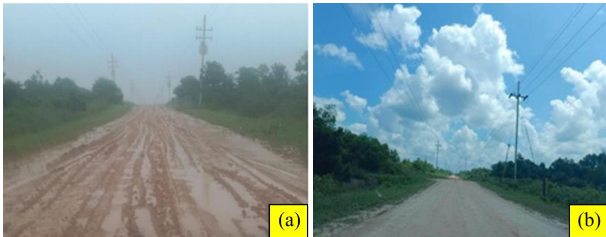
Figure 8. Field condition of existing soil stabilized with 5% cement and 1% chemical additive (before and after treatment)
