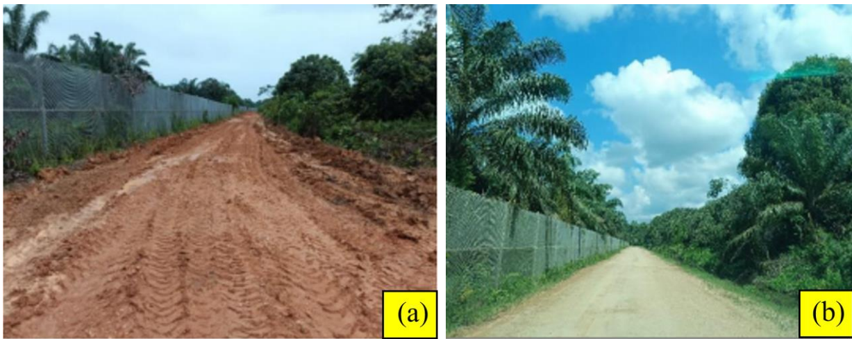
Figure 8. Field condition of existing soil stabilized with 5% cement and 1% chemical additive (before and after treatment)
