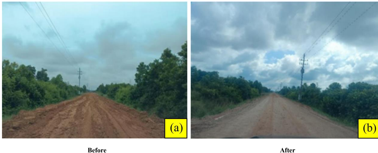
Figure 10. Field condition of existing soil stabilized with 5% cement, 1% chemical additive, and coarse aggregate 15 cm (before and after treatment)
