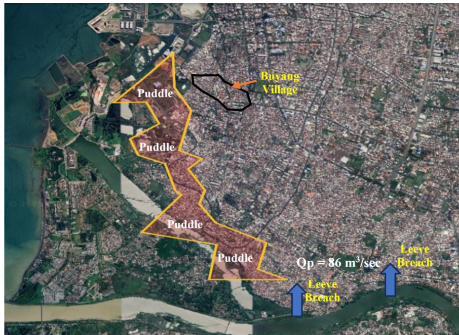
Figure 11. Flooding area caused by a levee breach
