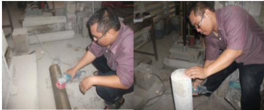
Figure 7. Leveling the test specimen for the installation of GFRP material
