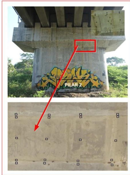
Figure 3. Around 120 retro targets attached to the pillar facade
