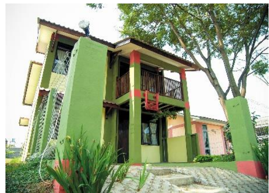
Figure 5. Two-story RISHA house
