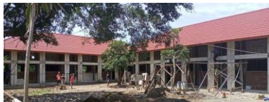
Figure 2. Construction Phase of Budibakti Elementary School Utilizing RISHA
