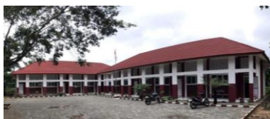
Figure 3. Exterior Photograph of Budibakti Elementary School Constructed with RISHA
