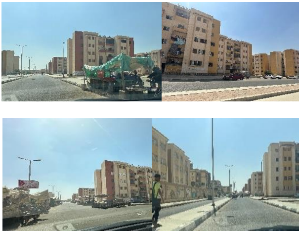
Figure 19. The general characteristics according to the quality of life indicators – Zone 8. Source. Researcher, based on the field visit
