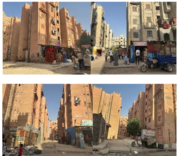
Figure 9. The general characteristics according to the quality of life indicators - Zone 3. Source. Researcher, based on the field visit
