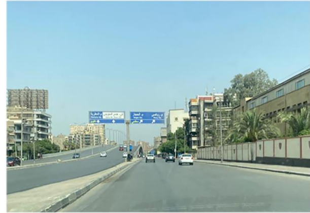
Mahkama flyover from Abu- Bakr EL-SediK - street
