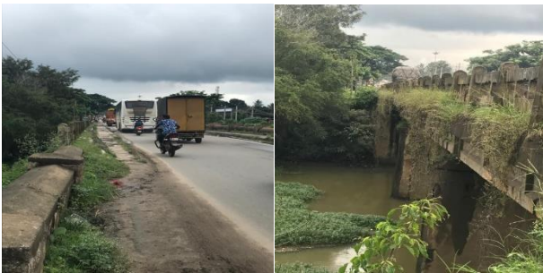
Figure 1. Bridge connecting Mysore and Hunsur-Madkeri Road
