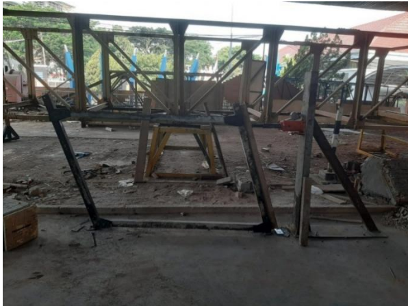
Figure 3. Testing of Steel Frames without Masonry
