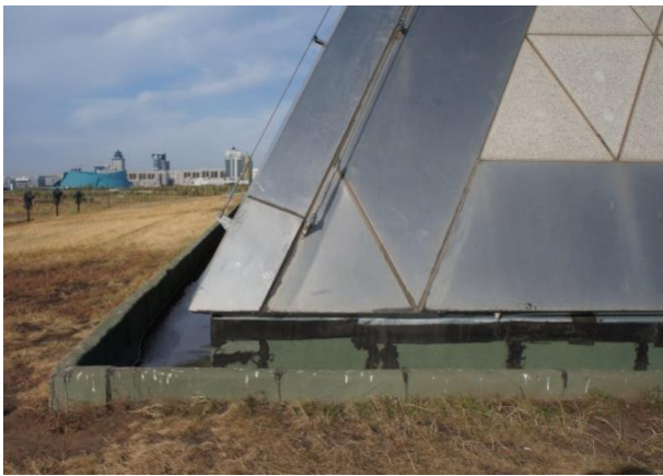
Figure 6. Assembled component of mobility of the Palace of Peace and Reconciliation building
