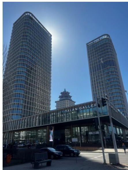
Figure 8. Talan Towers, 2017, Astana
