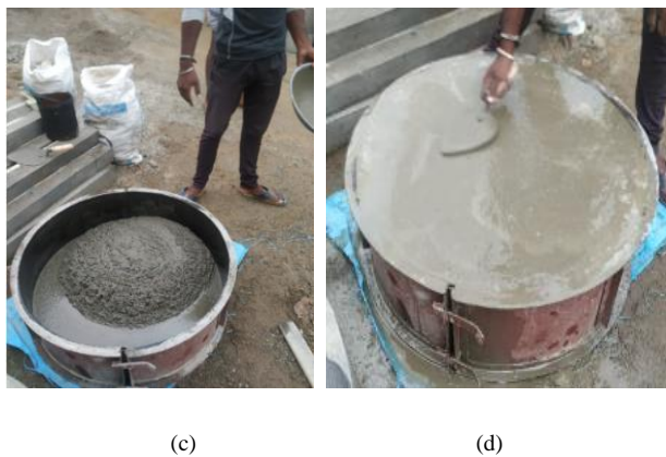
Figure 2. Foundation Block Casting (a)Initial Mound Preparation (b) Mixing of Concrete (c)Filling of Mould with Concrete (d) Completed Foundation Block
