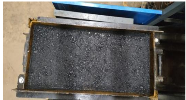
Figure 4. Surface Layer Construction
