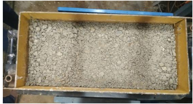
Figure 3. Sub Base Layer Construction
