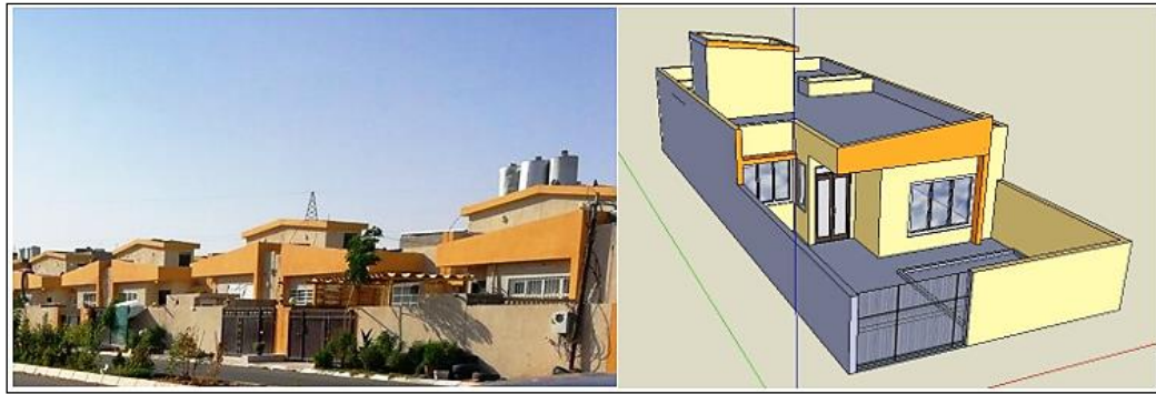
Figure 2. (Left) The selected row-houses facades in 'Garmian', 3D model for single typical row house. (By Researchers)
