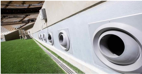
Figure 6. Nozzles alongside the pitch: Photo by [43]
