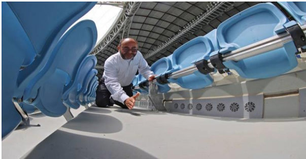
Figure 7. Dr. Ghani examines nozzles for cooling fan seats at Al Janoub Stadium: Photo by [41]
