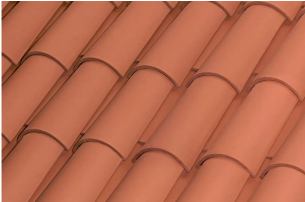
Figure 2. Clay Roof Tiles
