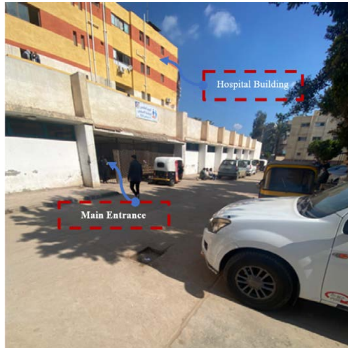
Figure 12. Main Entrance of Existing Hospital - researcher
