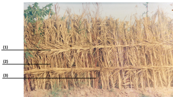
Figure 4. A traditional whole date palm leaves fence in Islamic Qasr Village. (1) A belt made from a whole date palm leaves. (2) Vertical whole date palm leaves. (3) An intermediate acacia logs post
