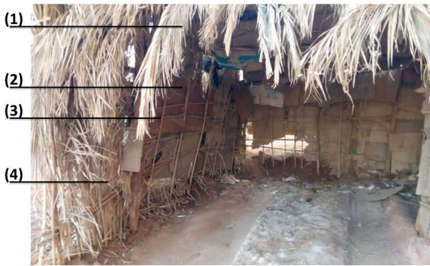
Figure 10. A garage made from leaves and cardboard in new Qasr town from the inside
