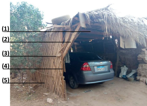
Figure 11. A garage made from timber frame and date palm midrib in new Qasr town. (1) A Casuarina beam. (2) A Casuarina overhang. (3) A horizontal date palm midrib belt. (4) Timber frame. (5) Diagonal midribs nailed to the timber frame
