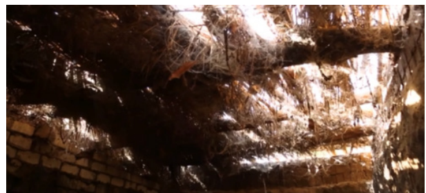
Figure 3. Date Palm Leaves in a traditional Shari'a roof in the Islamic Qasr Village
