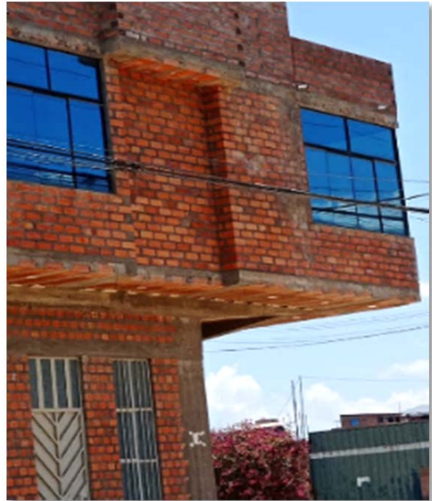
Figure 12. Abrupt changes in stiffness of floors
