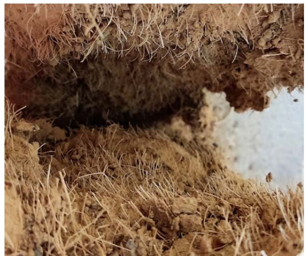
Figure 12. Fracture of the mass
