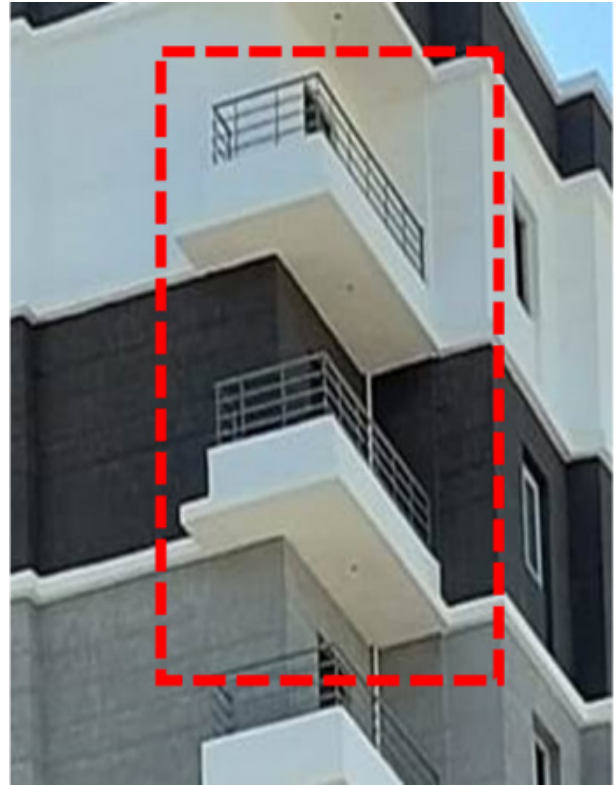
Figure 35. Corner of building [19].
