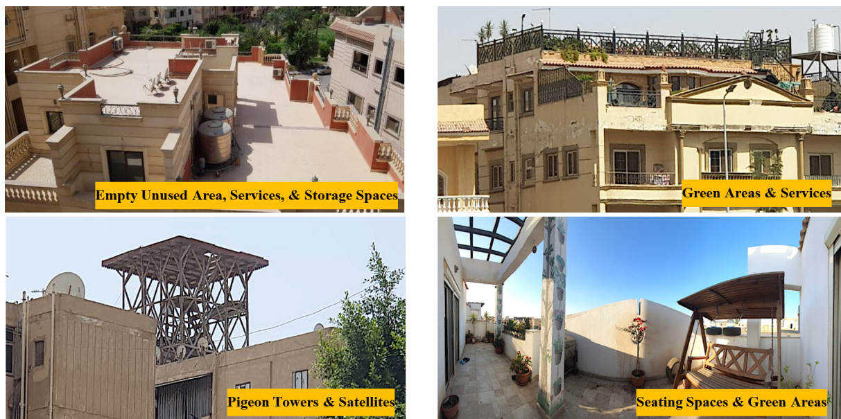
Figure 13. Samples of Residential Rooftop Patterns Use in New Cairo (Author, 2021-2022)
