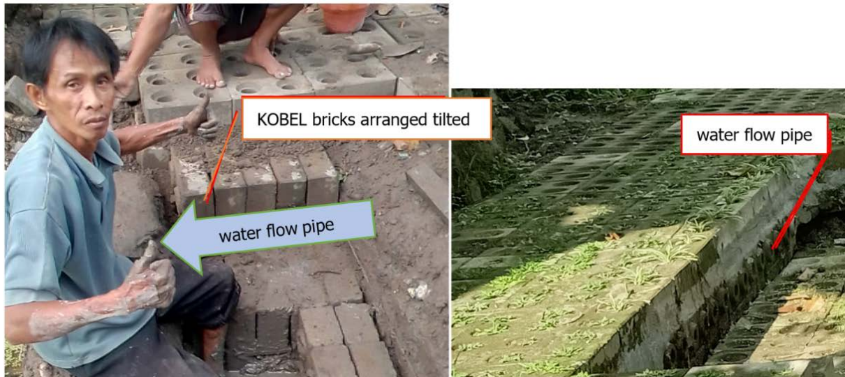
Figure 5. The use of KOBEL bricks as water flow and ground cover
