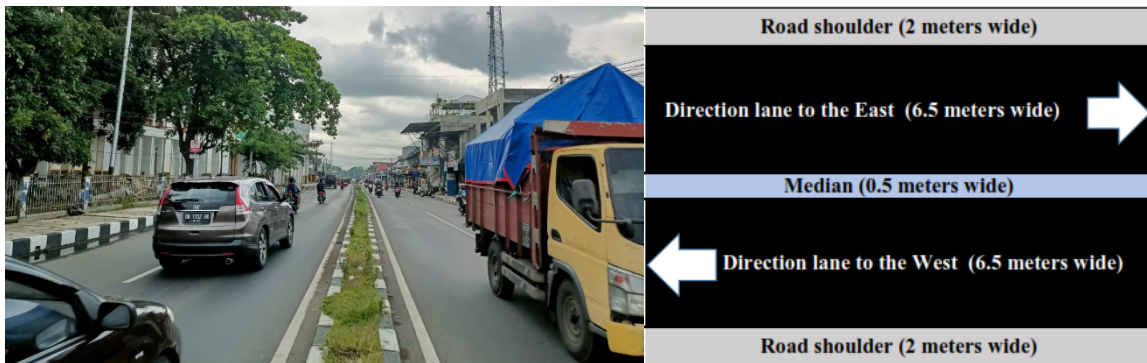
Figure 2. Section road condition with median type 4/2 D
