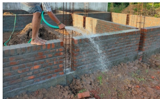
Figure 2. Typical RCC columns erection and curing activity
