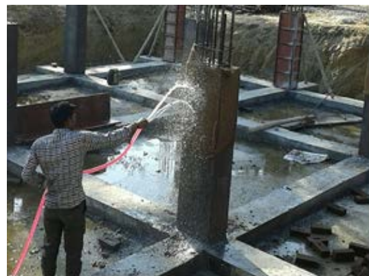
Figure 1. A typical scenario of excavation and foundation for small buildings
