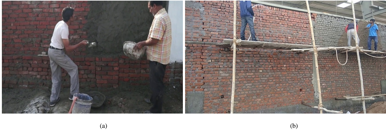
Figure 4. (a) and (b): A general method of cement plastering on brickwork
