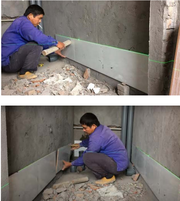
Figure 7. Laying ceramic tiles on toilet walls
