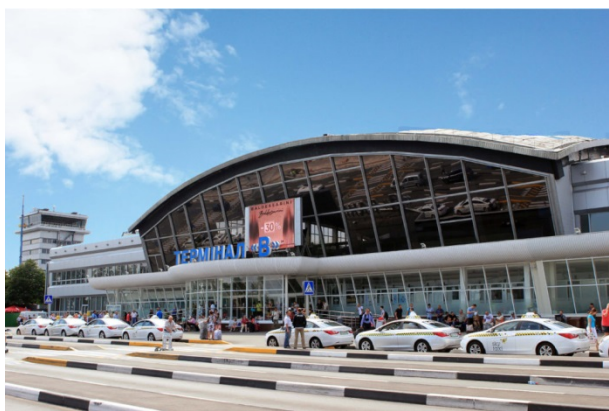
Figure 3. Boryspil International Airport (Source: https://kbp.aero/wp-content/uploads/2017/08/t1.jpg )
