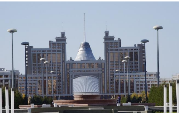
Figure 3. Complex of buildings of NC KazMunayGas JSC. Astana
