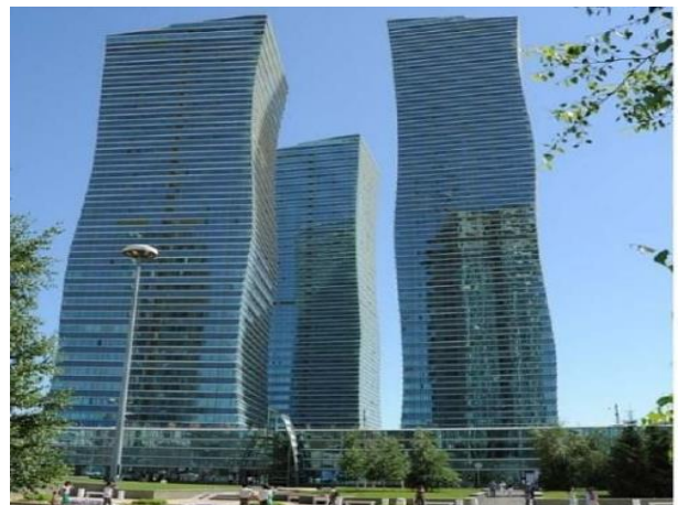
Figure 12. Northern Lights complex. Astana
