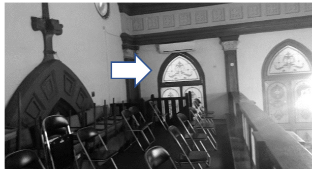
Figure 6. Northwest Balcony Conditioning Location
