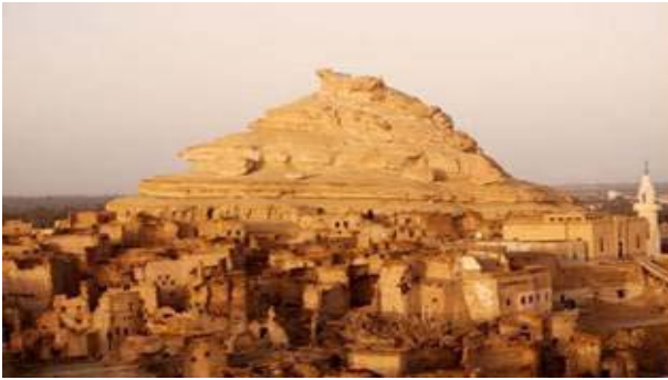
Figure 3. Mud houses of Siwa town in Egypt [17]
