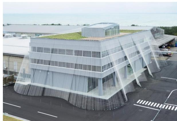
**Figure 13.** Earthquake-Resistant Building Made with Carbon Fabric [14]
