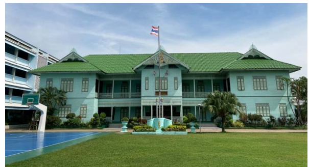
Figure 6. Namphetch building, Nareerat school, Phare, this building was built in 1921.
