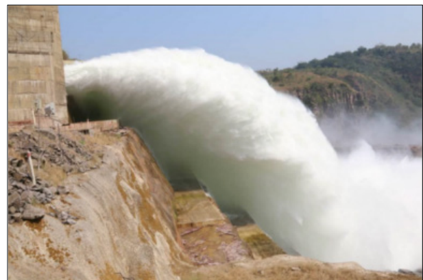
Figure 3. Picture of the flow passing over the spillway-flip bucket system
