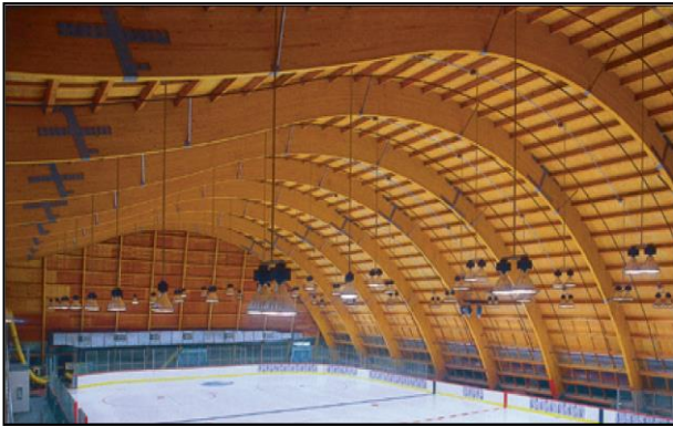
Figure 1. The Disney ICE rink in Anaheim, California Features Glulam Arches Curved to a 75-Foot Radius to Form The Ice Center's Roof System.
