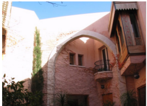
Figure 9. Al Tabbaa Villa: Balconies overlooking each other's and outlook view inner courtyard. Also, to achieving a balanced economy and simplicity.
