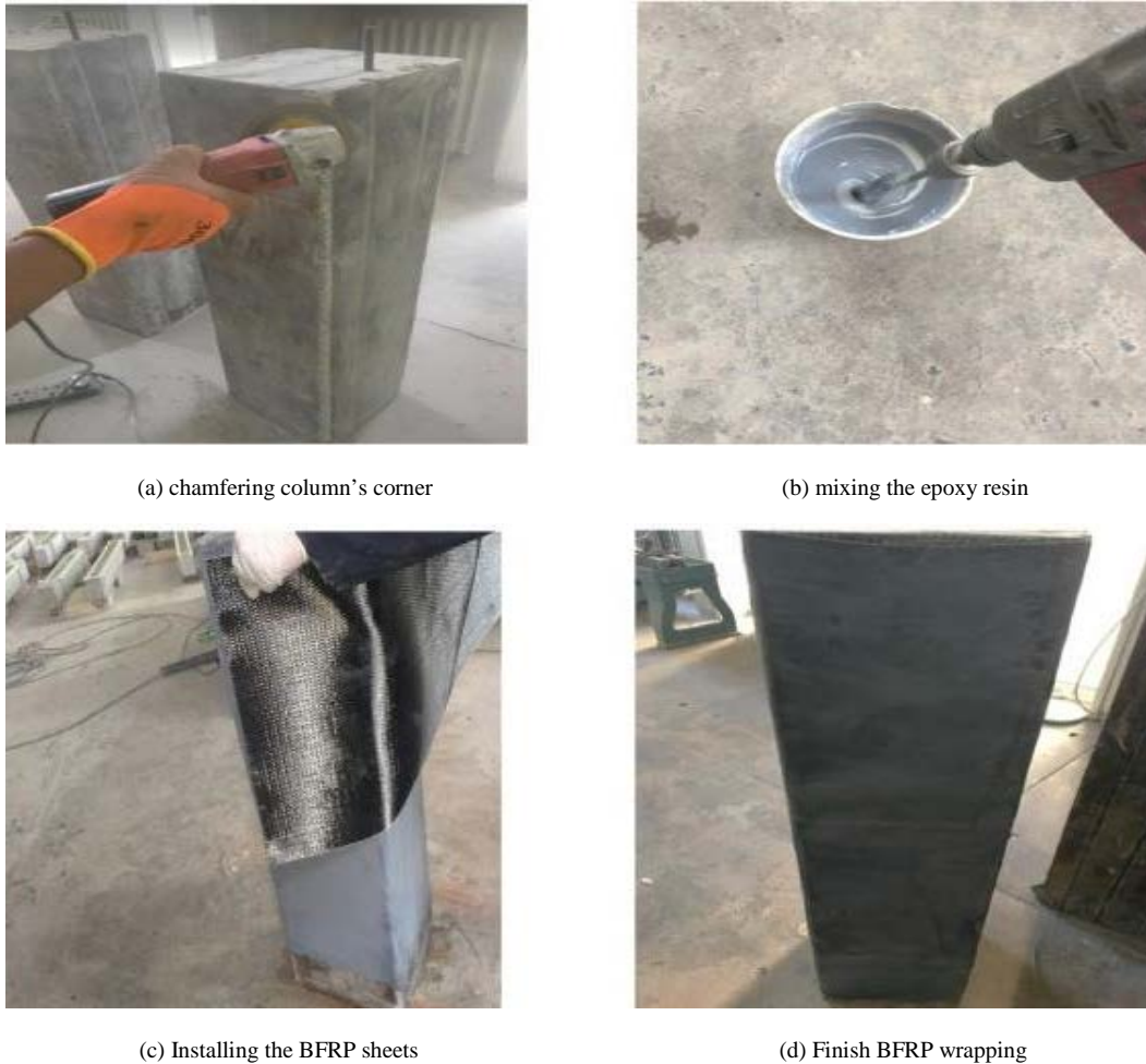
Figure 4. Repairing process using BFRP sheet
