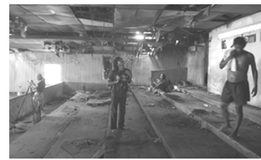
(3) Surveying Saowapa Rama theater, June 5th, 2012
