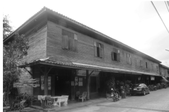
(2) Building no.2: a wooden two-story row house, built in 1941
