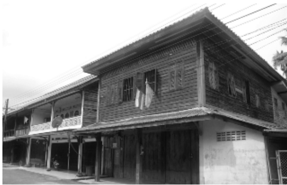
(3) Building no.7: Mrs. Prayad Boonyasit's house, built in 1940
