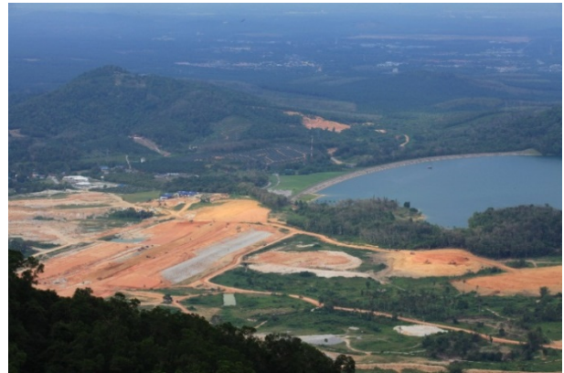
Figure 1. Overall view of the Mengkuang Dam during construction (CFWong, 2012)
