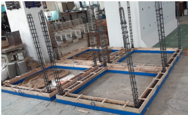
Figure 7. The process of reinforcement
