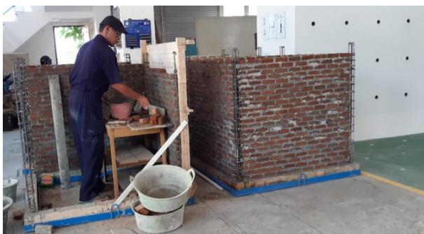
Figure 8. The process of wall construction
