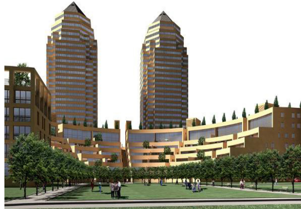
Figure 14. "Towers" housing complex, Dnipro, Ukraine
